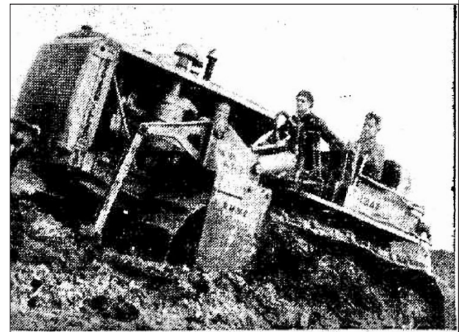
A big bulldozer battles with mud, making a path for a direct rail link with Yallourn.
