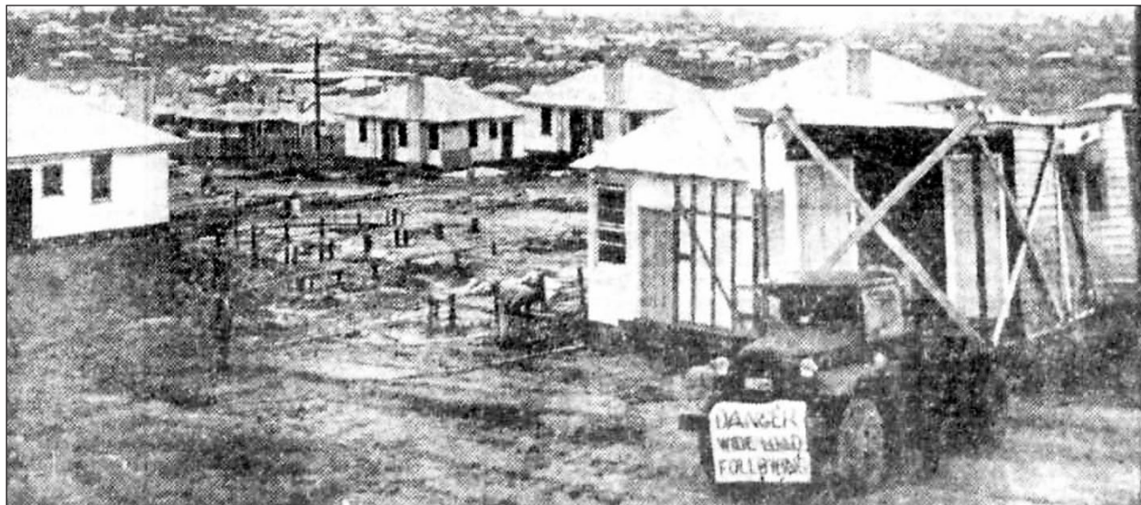
Prefabricated homes being unloaded on the Housing Commission estate. Approximately 200 homes have been built in this area and 250 more are under construction.
